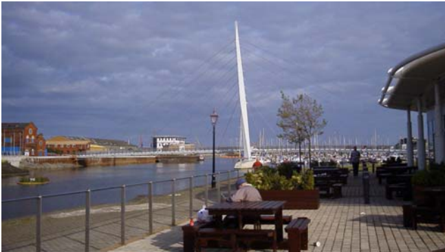
Fig. 26: Port Tawe Footbridge
