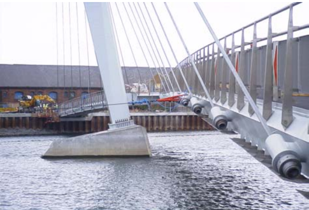
Fig. 29: Port Tawe bridge deck
