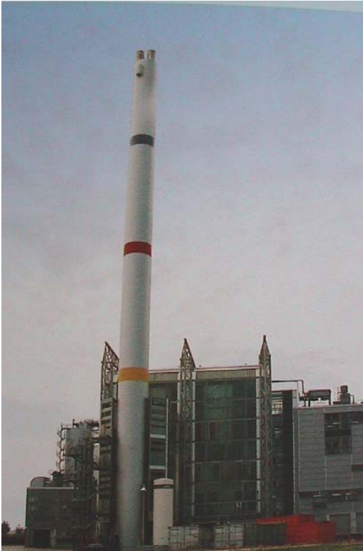
Fig. 36: MH-Power Plant Ulm - Germany
