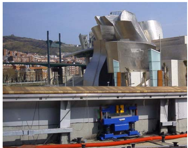
Fig. 22: Installed MTMD-V in bridge rail
